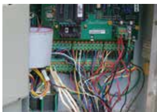
Circuit boards receive signals that in turn open the underground valves to the sprinkler heads!
